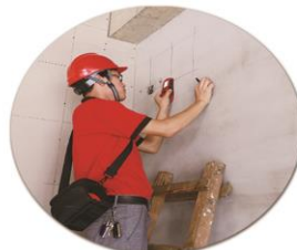
Installation of furniture and air-condition.
