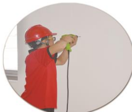
The location of rebar for drilling, cutting and coring operations
