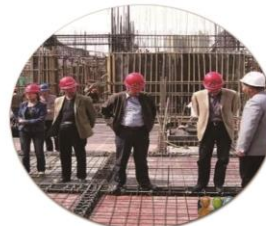
Inspecting and accepting concrete structural construction quality.
