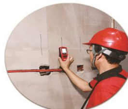
Testing the distribution and direction of electric cables, pipelines and metalwork inside walls and floors.
